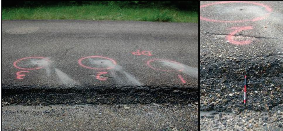
Figure 23. Use of a combihammer to drill holes in asphalt for density probe insertion.
